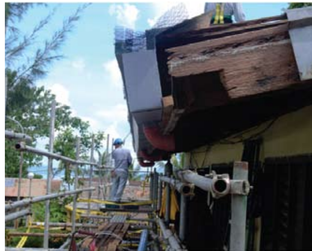
FILTERS WERE INSTALLED TO PREVENT GUTTERS FROM CLOGGING
