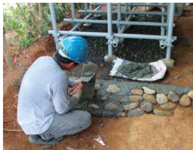
A PROJECT EMPLOYEE WORKING ON THE RESERVOIR'S FOOTING
