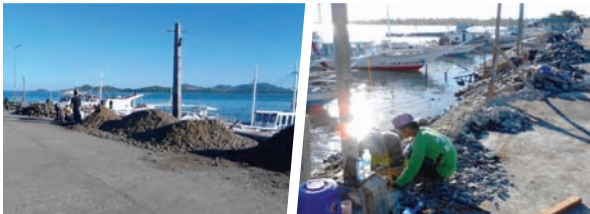
Bancal Wharf Rehabilitation
